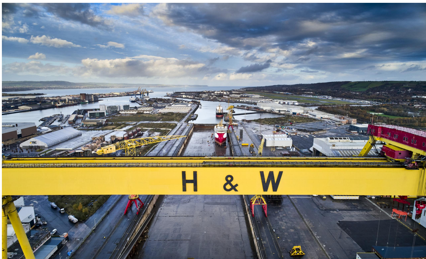
Harland & Wolff Shipyard building dock. Photography by davidcordner.com
